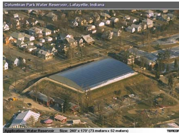
Columbian Park Water Reservoir, Lafayette, Indiana Application: Water Reservoir Size: 240' x 170' (73 meters x 52 meters)
