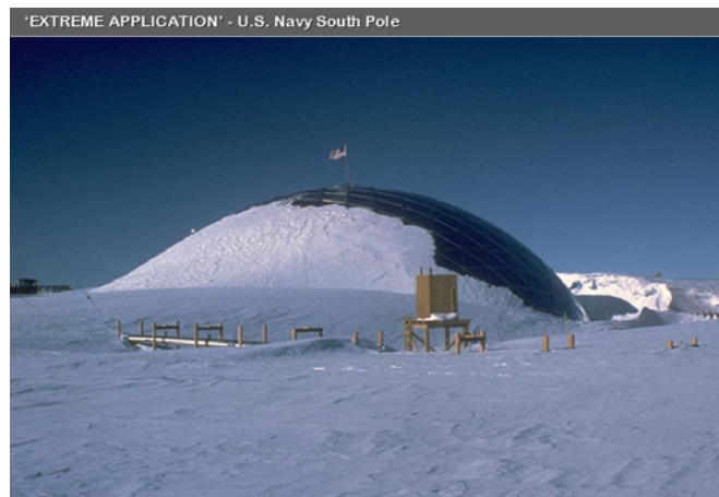
50 m (164') diameter designed for 1465 kg/m 2 (300 psf) snow load
